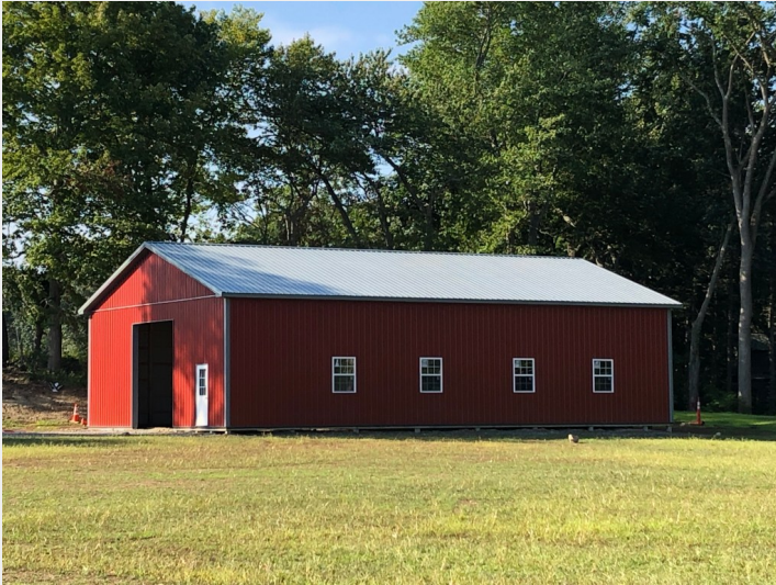
New Pole Barn at Easton's Volunteer Firefighter's headquarters. - Photo by Rick Falco
