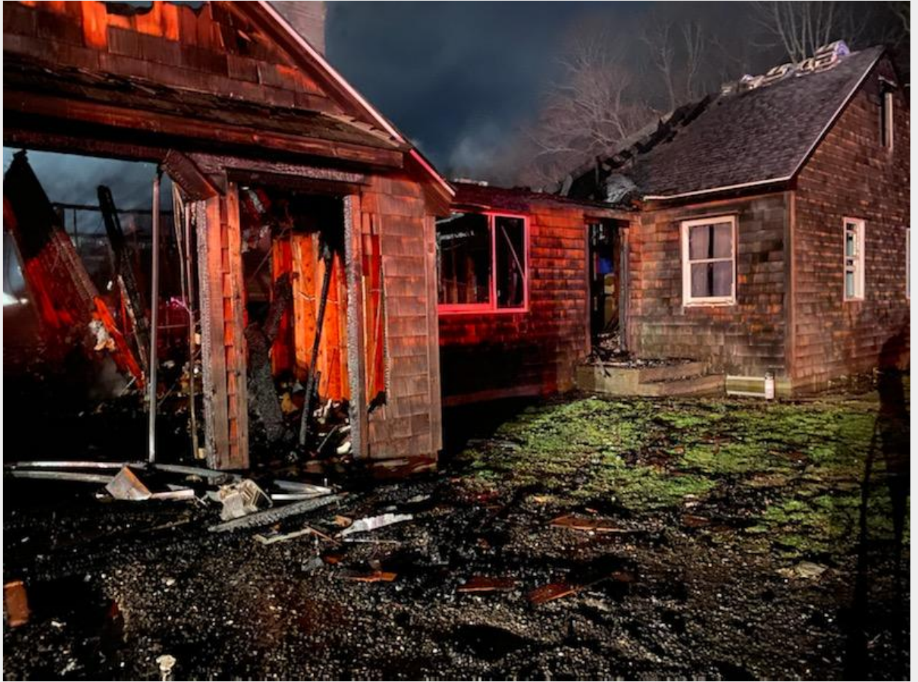
• The house at 330 Rock House Road is inhabitable. — Photos Courtesy of Easton Fire Department
